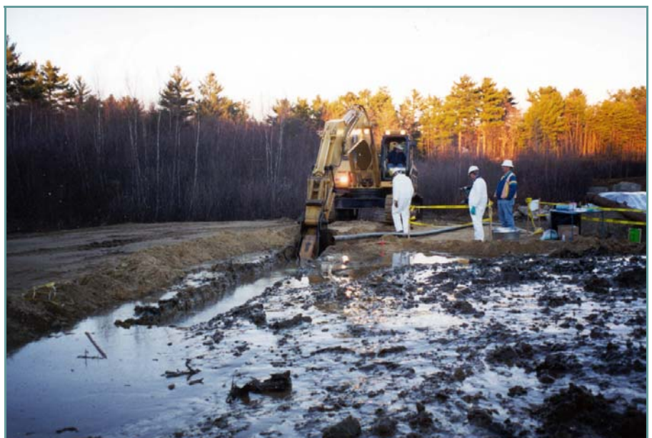
Pilot-Scale PRB Installation using Biopolymer Slurry Trench, Somersworth, New Hampshire
