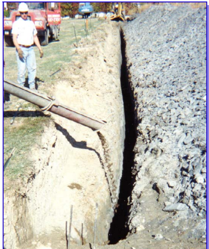
PRB Construction in Cleveland, Ohio
