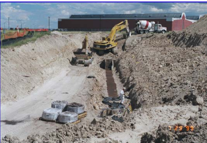
Permeable Reactive Barrier Construction at F.E. Warren AFB, Wyoming July, 1999
