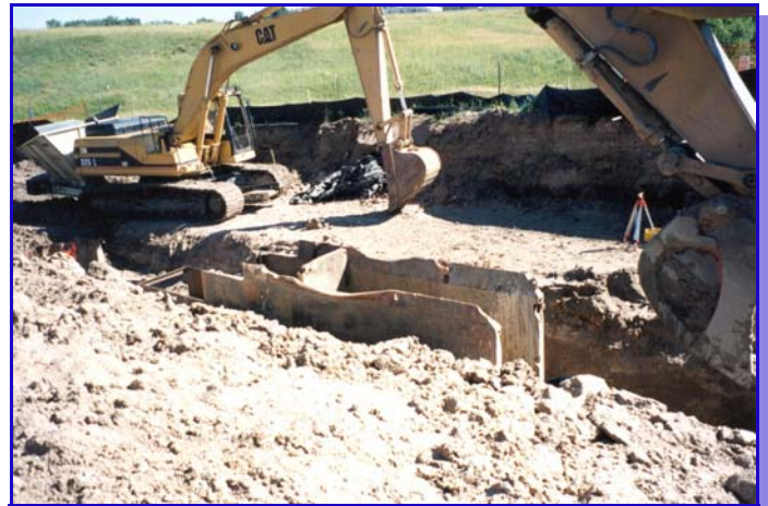
Trench Box Excavation at F.E. Warren AFB, Wyoming July, 1999
