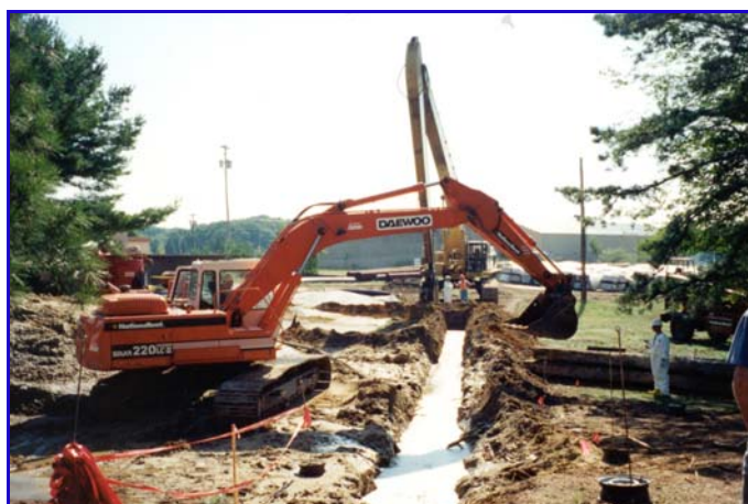
BioPolymer Trench Excavation at Pease AFB, New Hampshire August, 1999
