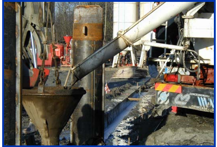
Iron Placement through a Tremie Pipe
