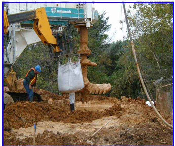
ZVI-Clay Zone Installation, Martinsville, NC
