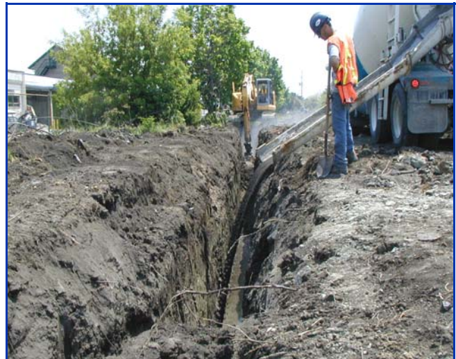
Iron PRB Placement in Toronto, Ontario
